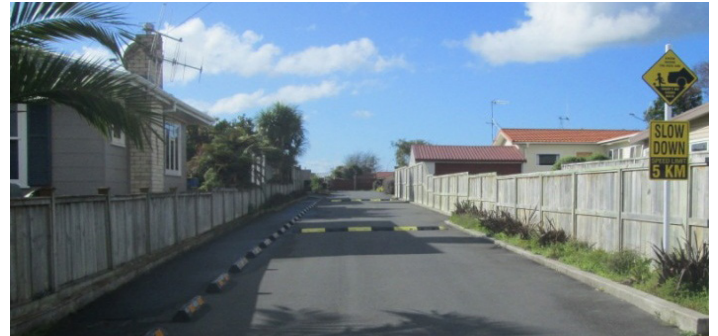
This long driveway has been made safer with speed bumps and a separate pathway for pedestrians.
