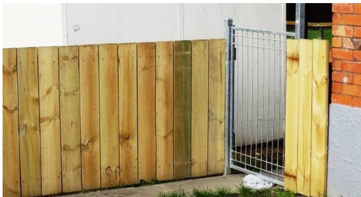
We are installing secure fences like the one above to separate play areas from driveways.
