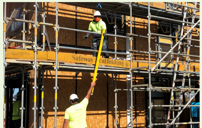
Safety comes first at Precision Construction work sites
