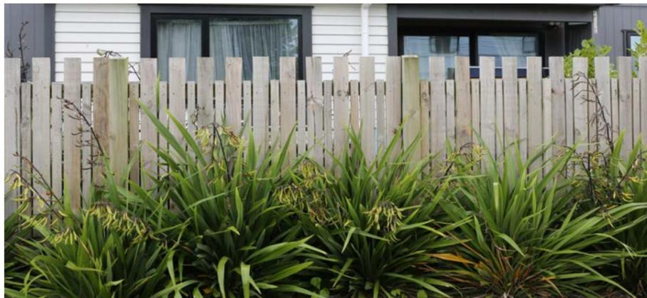
1200mm timber batten fence along a common accessway.
