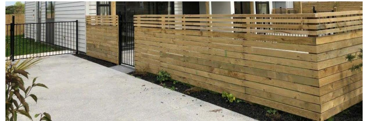
Horizontal slatted timber fence with a 300mm permeable top.
