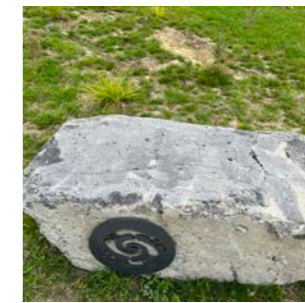
Kowhatu (basalt) wayfinding markers: A cost-effective and high-impact wayfinding solution. Can be used as large bollards along pathways and within garden beds. Note loose basalt will need a concrete footing or haunching to prevent movement.
