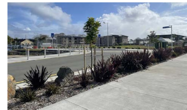
Ōwairaka's new Park edge road. Brush concrete finish with standard concrete mix and oxides can be used for all main courses of concrete paths.
