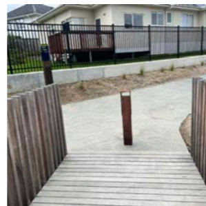
For all boardwalks, decks and bridges its encouraged to only use pine timber for the decking.
