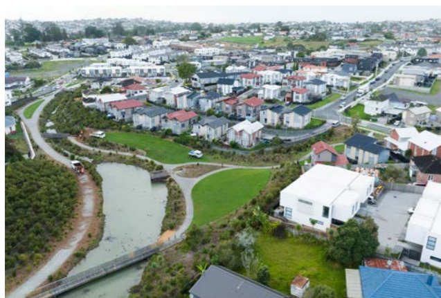
Freeland Reserve, Roskill South is designed to accommodate large rain events
