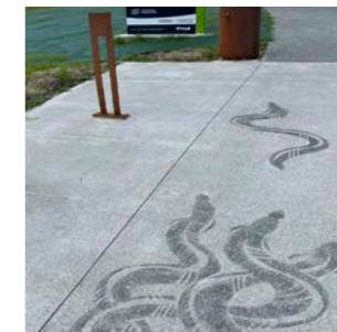
Stencils: An affordable and visually striking option for wayfinding. Stencils can be etched into concrete pavements and be suitable for other elements such as timber vertical markers
