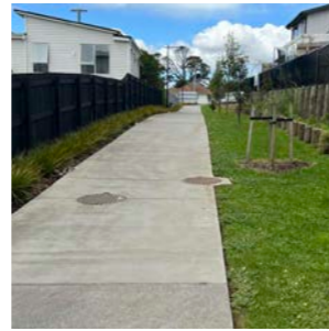
Standard concrete finish should be specified for all main courses of concrete for walkways within a park and public pedestrian pathways along the street.
