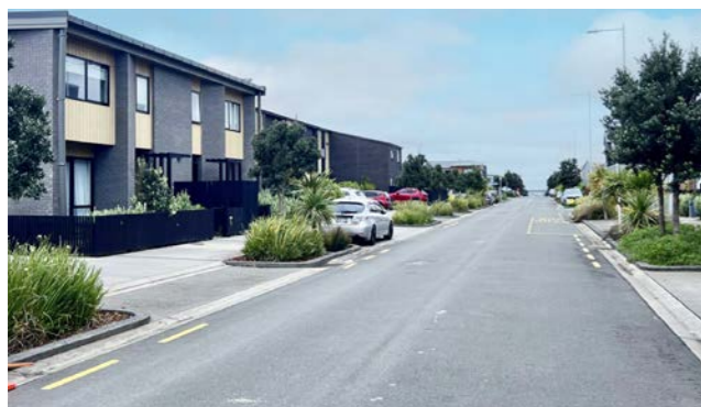
Wallace Road, Hobsonville. Large streets are the default option for new streets with buses and shared paths
