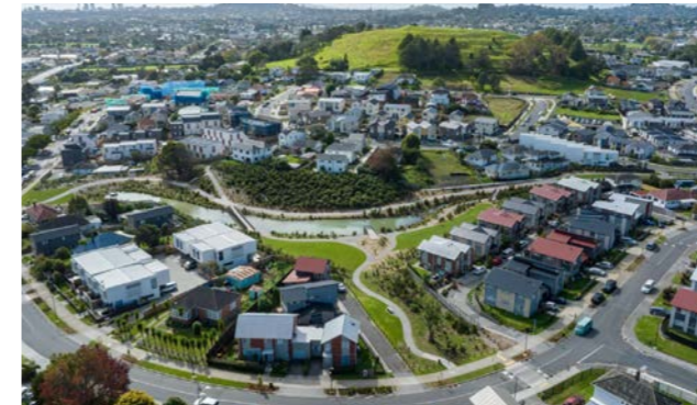
Freeland Reserve, Roskill South serves as a detention basin for large flood events when not used as a park
