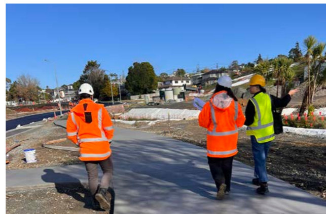
Maintenance and fair contract agreements need to be agreed between the asset owners at the outset of a project
