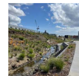
Stream daylighting at Te Ara Awataha, Northcote
