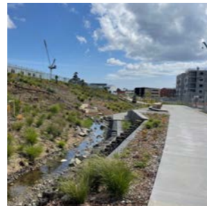
Pathways along esplanades, water courses and areas prone to flooding can have an exposed aggregate concrete finish to add extra levels of slip resistance.
