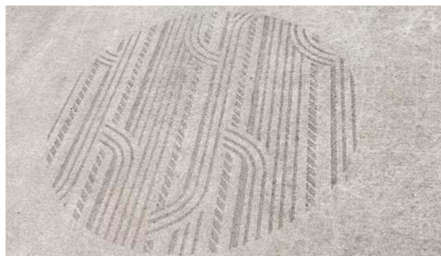
Stencil artwork on concrete pavements is a good way to provide wayfinding and a cultural narrative at a low cost
