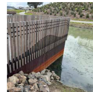
Steel bridge with artwork
