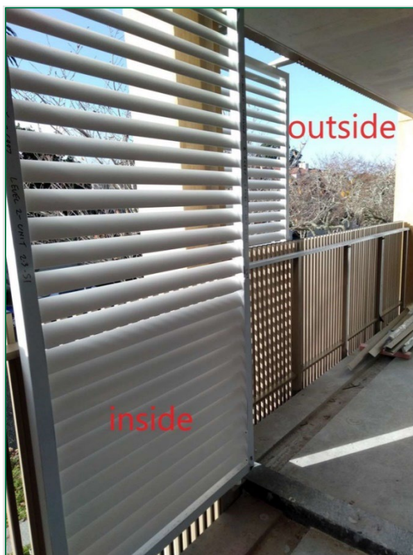
Figure 7: Privacy screens located on the inside and the outside of a balcony
