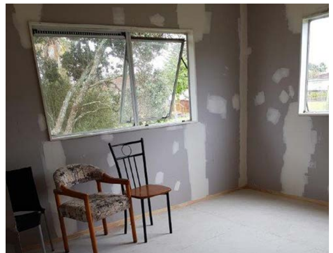
New walls and floors at the property
