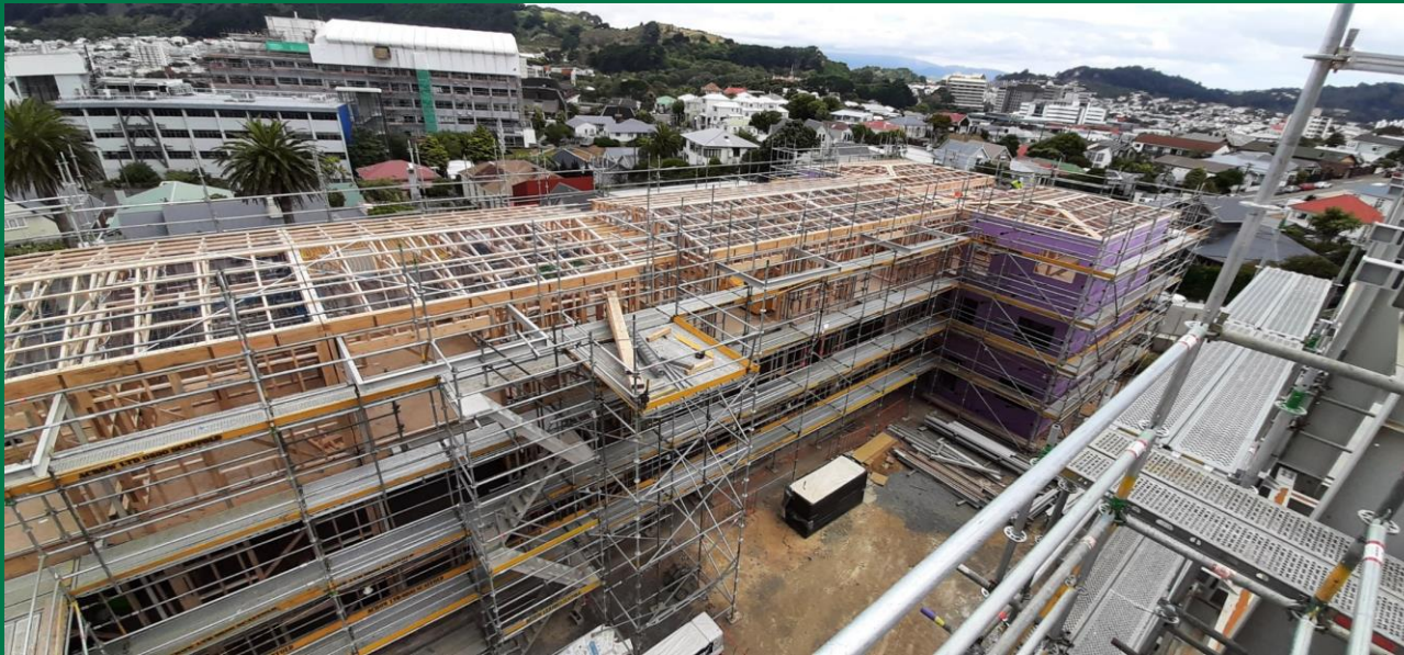
Block C roof structure complete, and GIB weatherline being installed
