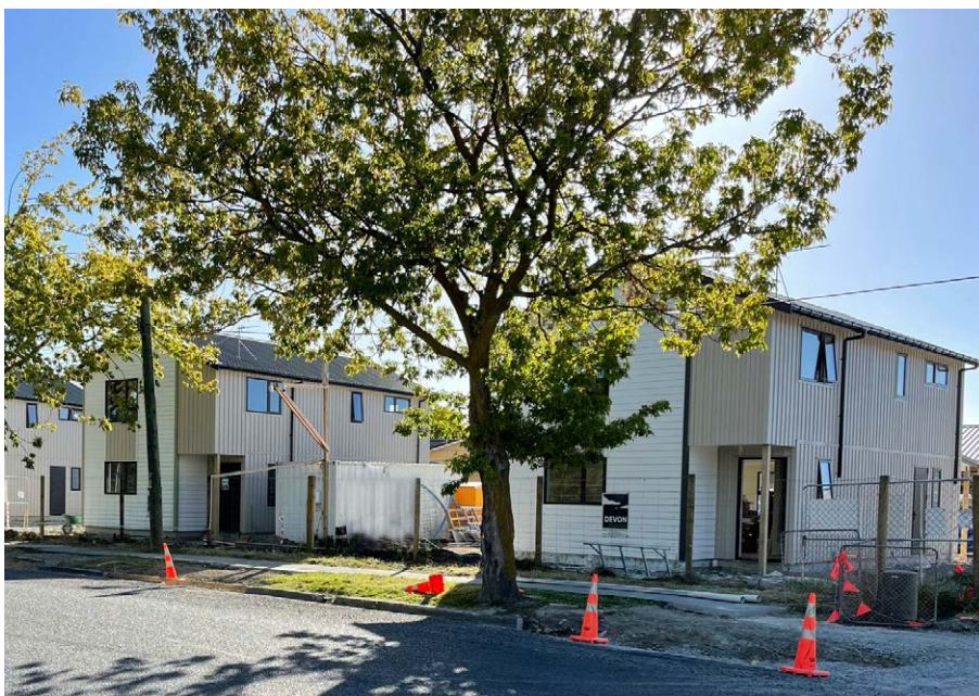
Family homes that are nearly complete at Bledisloe Road
